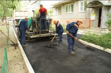
A photograph showing several workers in blue uniforms and hard hats working on a paved area in a courtyard. They are using tools like rakes and brooms to finish the surface. A concrete curb is visible in the foreground. |
