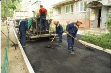
A photograph showing several workers in blue uniforms and hard hats working on a paved area in a courtyard. They are using tools to finish the surface of a new driveway.                  |
